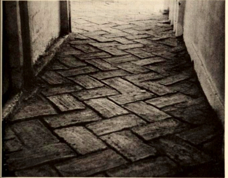
◇ Brick floor in arcade (low-cost experimental housing, Mexicali)
