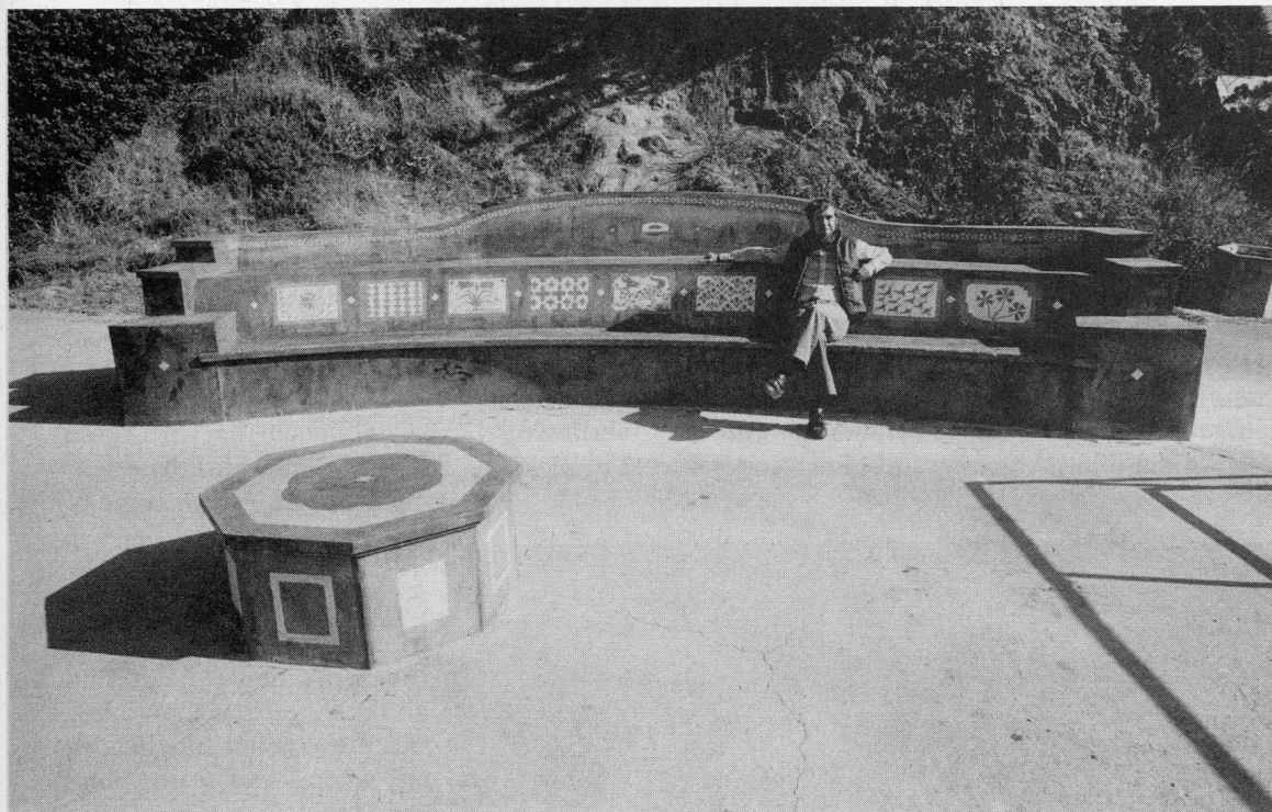
An uncommon bench collaboratively designed by Christopher Alexander and 23 friends. The objective was to make an ornamental seat that would be something worth fighting to save in 100 years. Made of poured concrete with inlaid green and white terrazzo decorations. About 20 feet long, it's four feet high at the crest.
