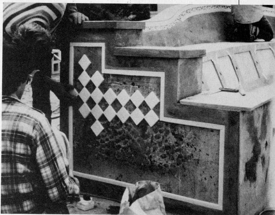
Dave Depper and Chris Berendes glue white diamonds of styrofoam onto the bench end. Terrazzo, a mixture of cement, marble dust, marble chips, and, in this case, green pigment is packed into the recessed areas. When it hardens the foam is picked out, and white terrazzo is packed into the remaining areas.
